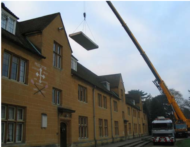
December 2004 - Removing the OCEES Building
