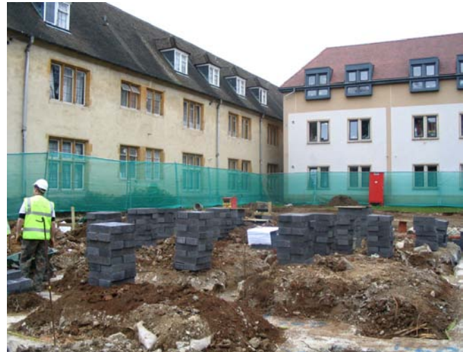
January 2005 - Building work begins
